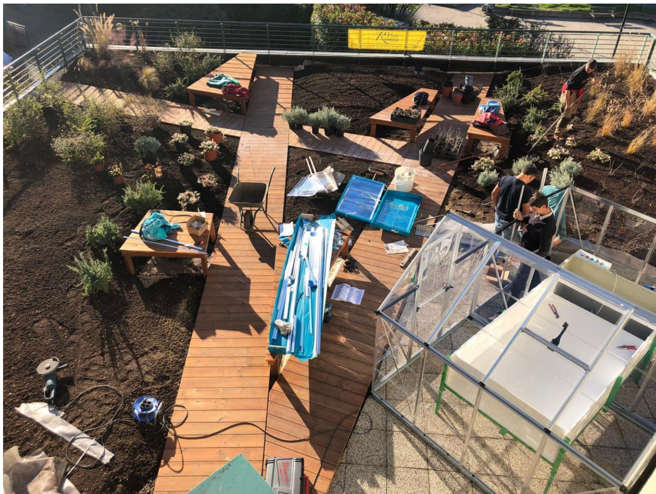
The green roof and the greenhouse
